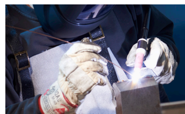
WIG welding process
